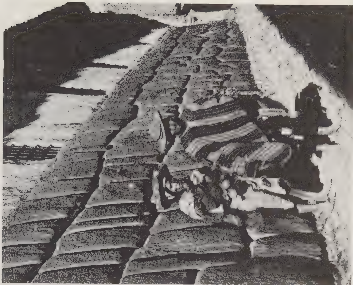
Cyclopean masonry of ancient Inca ruins, used here as the foundation for a relatively new building.
